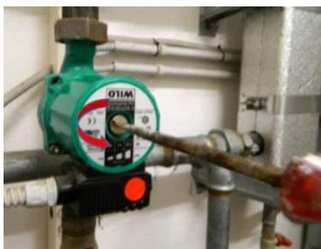
With a large screwdriver unwind the cap.
