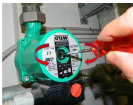
Then with a smaller one you can move the rotor of the circulator left to right that acts on the slot accessible under the removed cap.
